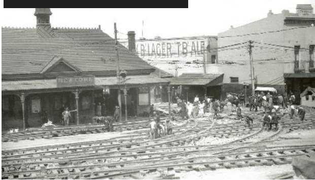
Laying new tram tracks.....
